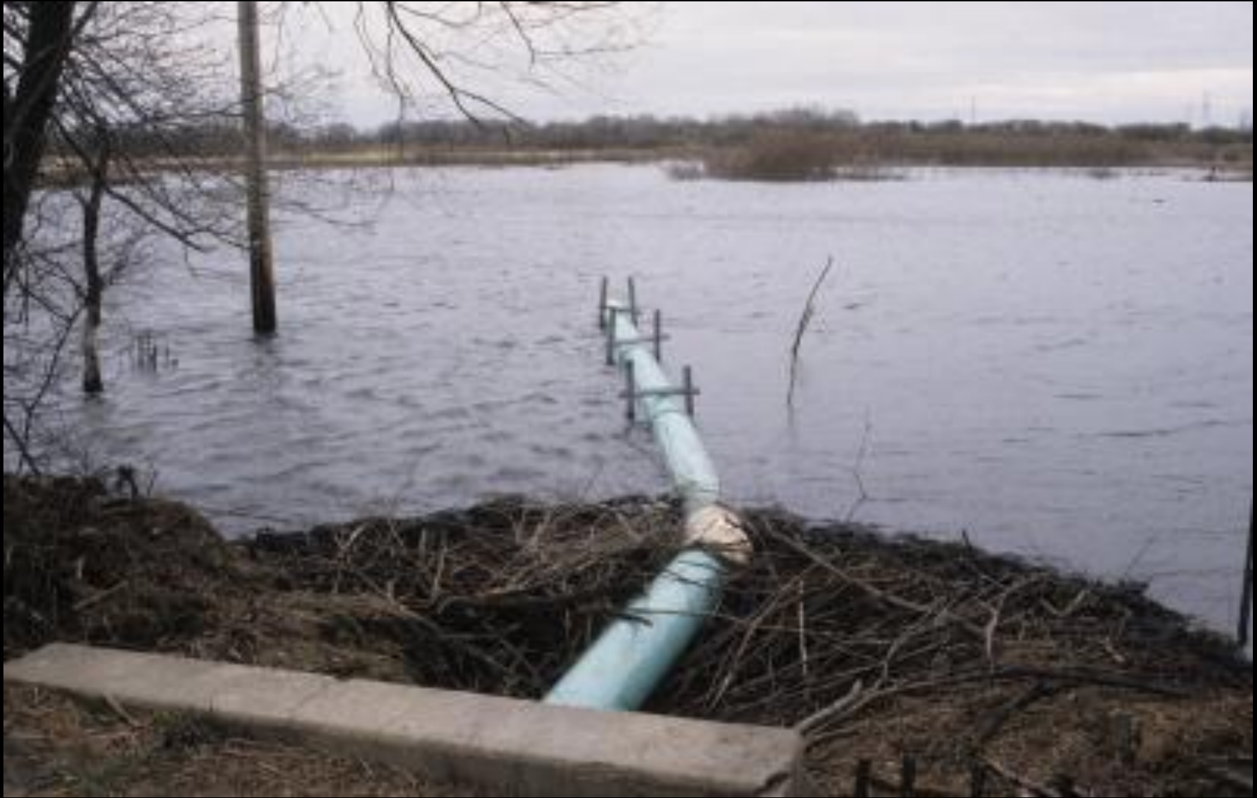
Water Control Device
