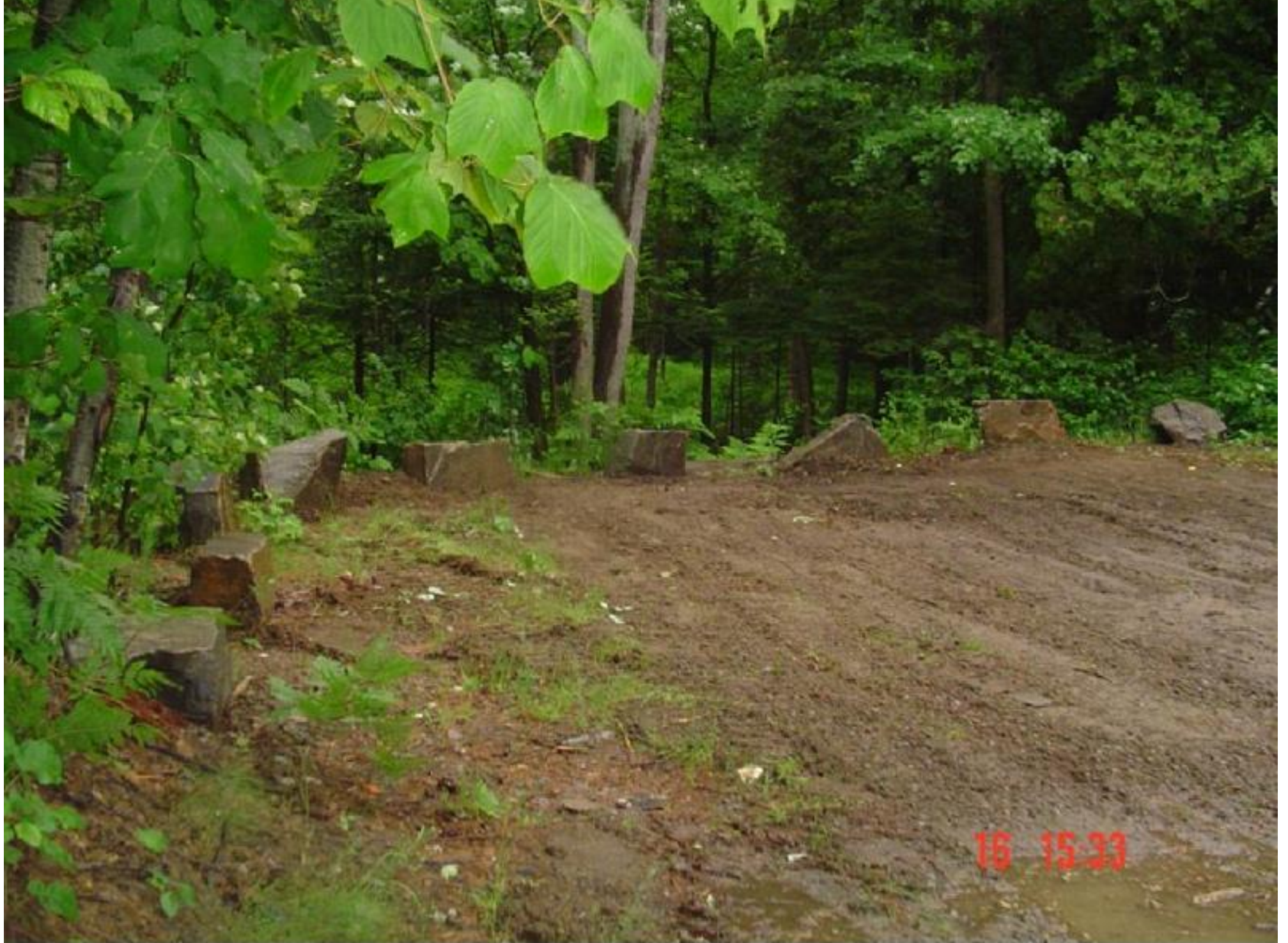
Armour Stone Stream Protection, Back of Parking Area
